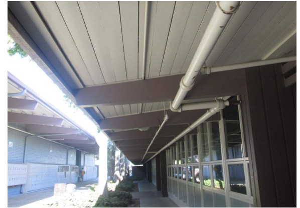
Exterior soffit condition with exposed sprinkler pipes
