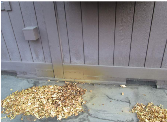
Splash damage at portable
