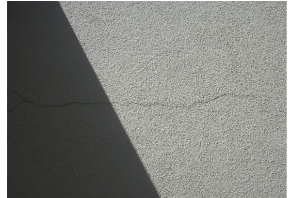
Minor plaster cracks
