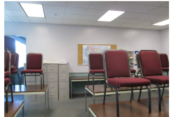
Classroom cabinets not secured to walls
