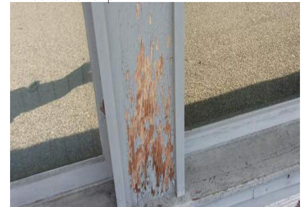
Damage at upper clerestory window
