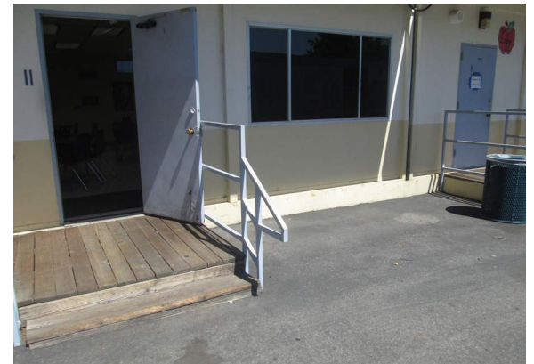
Ramps and Stairs in poor condition
