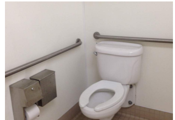
Water closet flush handle on wrong side
