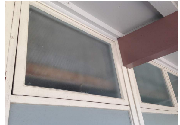
Single-pane windows with translucent glazing
