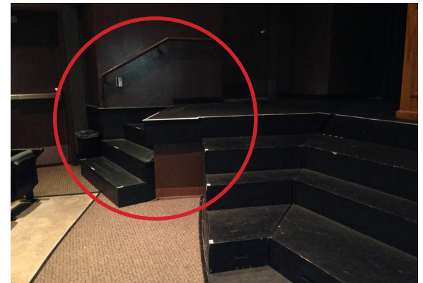
Non-compliant stair and railing at stage access
