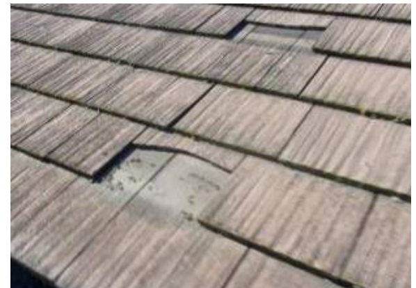
Damaged/missing shingle
