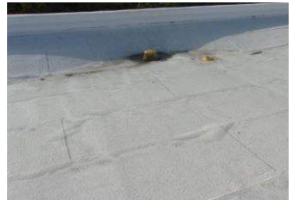
Blistering and minor ponding present at the roof
