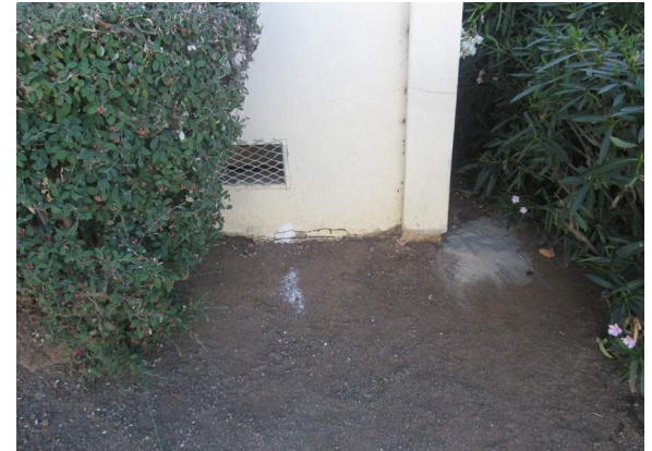
Inadequate grade separation
