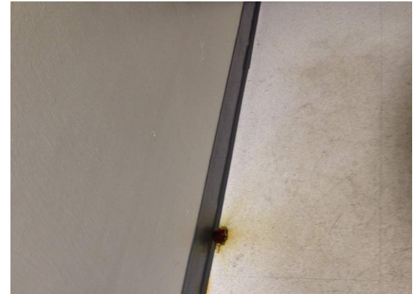
Condensation Drip at MDF
