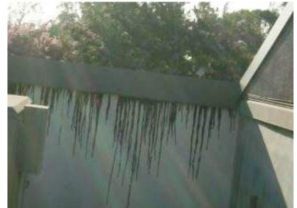
Parapet mastic in need of repair
