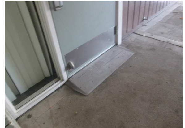
Threshold/entry ramp
