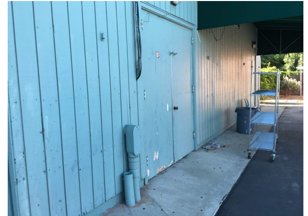
Deterioration at doors and siding
