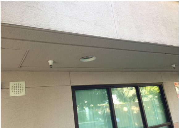
Building soffit - minor water stains
