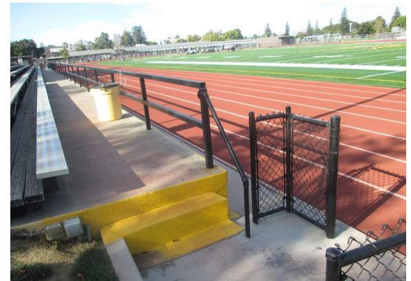
Non-compliant guardrail at front of bleacher walkway. No ADA seating areas provided.
