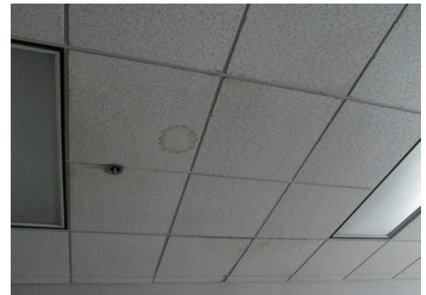
Damaged/stained ceiling tiles
