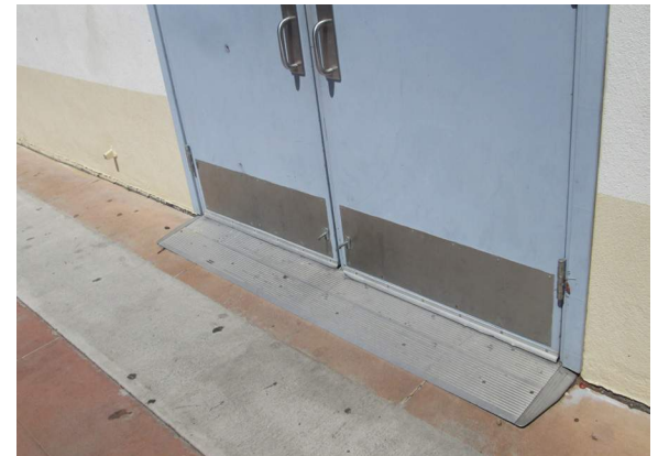
Entry slab subsidence
