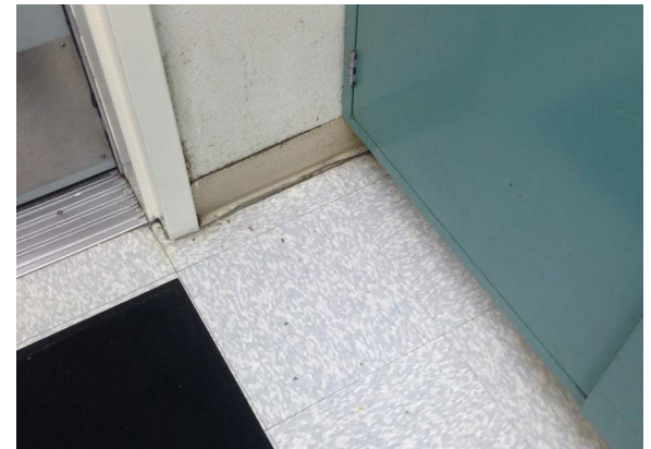
Staining at walls, floors and base
