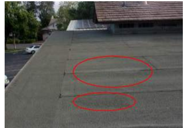
Blistering roofing cap sheet
