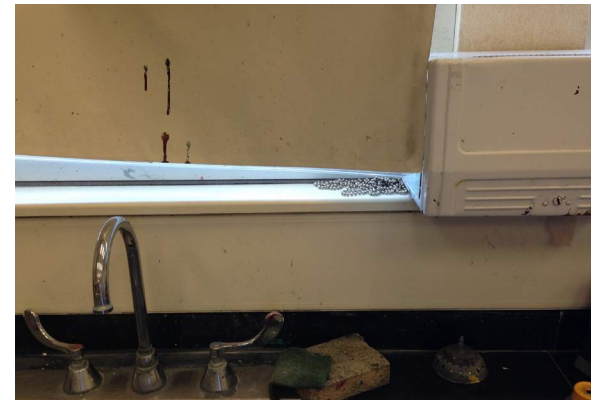
Paper towel dispenser inhibits proper mounting and operation of window shade. Damaged pull chain
