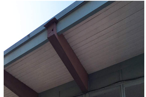
Deterioration at overhangs
