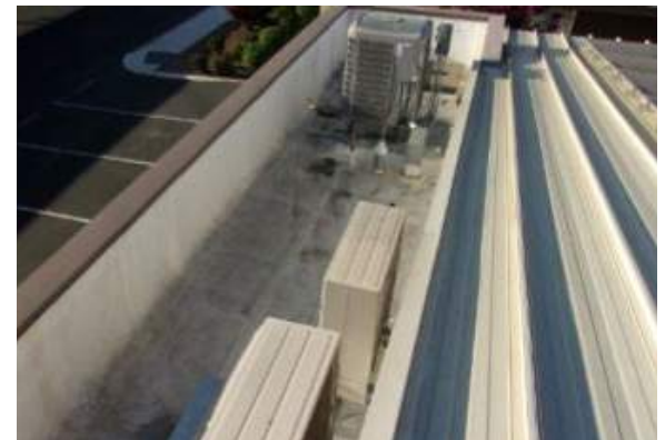
Built-up and standing seam metal roofs
