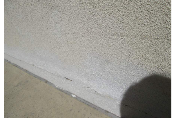
Damaged plaster at grade
