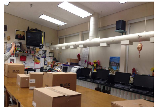
Low hanging ductwork
