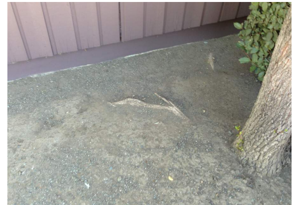
Tree roots growing close to building foundation
