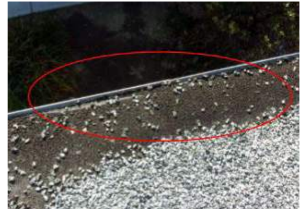
Exposed roofing piles
