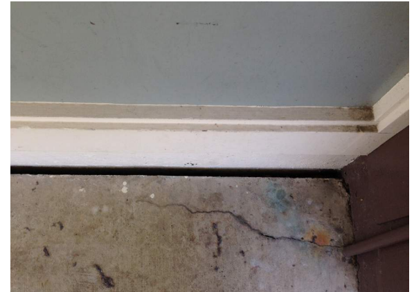
Exterior of Building- Sealant missing
