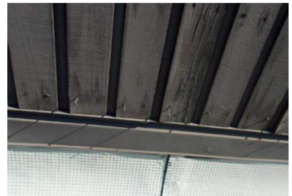
Loose fasteners at siding
