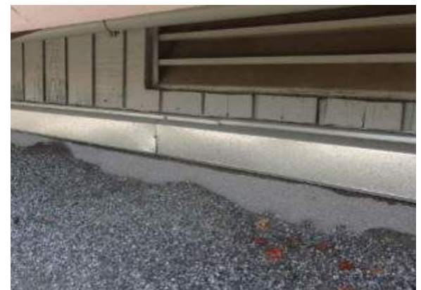
Damaged siding at upper roof sidewall
