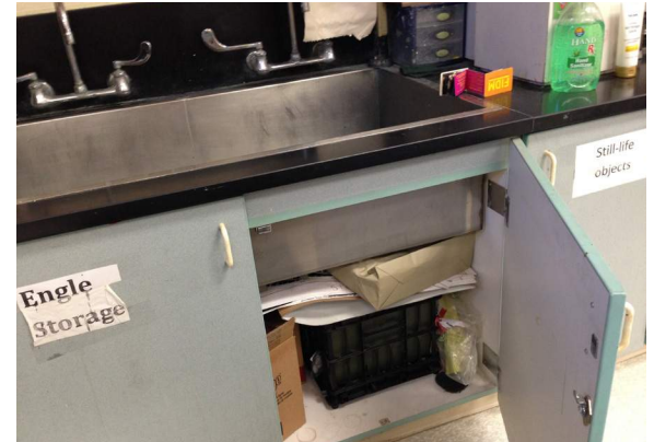
Cabinet base (non-removable) and sink depth do not allow for ADA access
