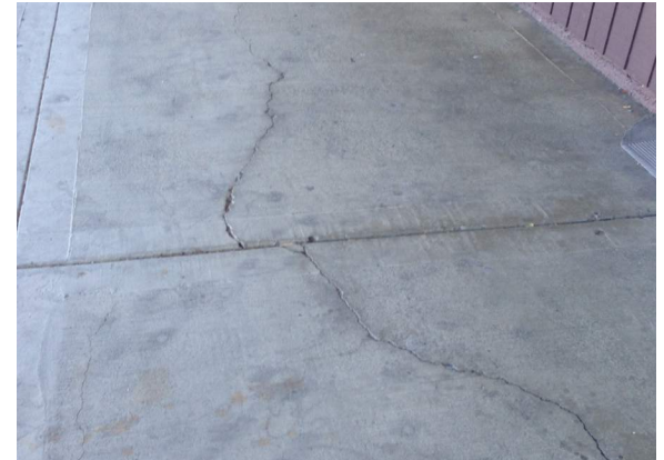
Cracking at walkway surfaces
