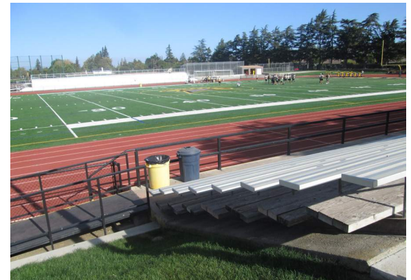
Non-compliant ramp railing and missing guardrail at sides of bleachers. Deck boards deteriorating
