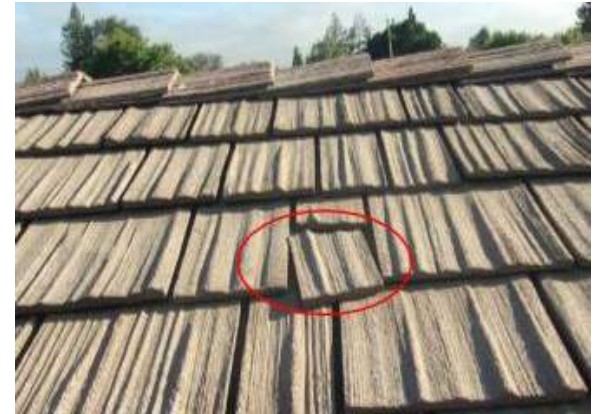
Damaged/missing roof shingles
