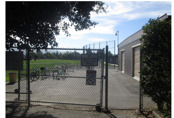
Non-accessible path of travel due to surface change
