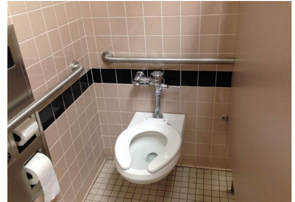
Dated finishes. Improper installation of grab bar/ toilet partition
