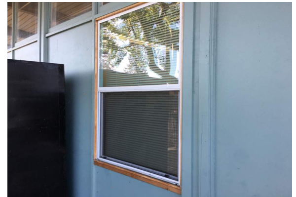
Window repair- untreated wood
