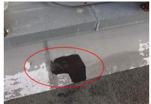
Weathered flashing at roof
