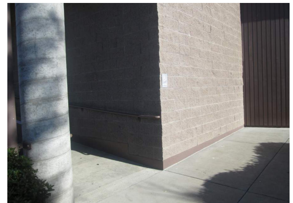
Railing does not continue beyond sloped ramp
